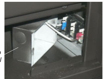
Remove cover to access Terminal Block
