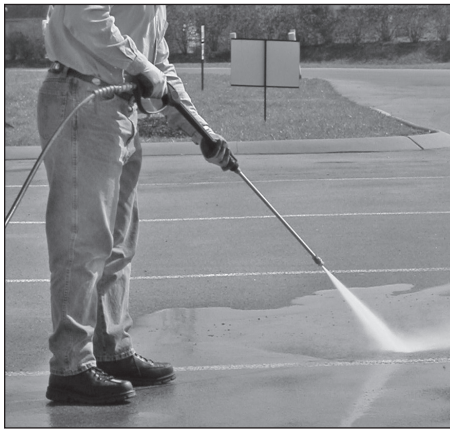
Figure 12 - Optimum angle to cleaning surface
