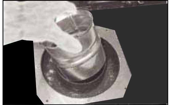
Figure 8.2 Remove the inner collar adapter.
