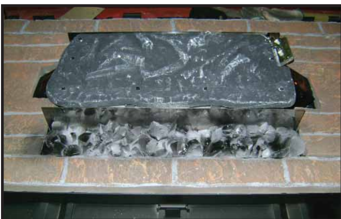
Figure 14.21 Finished Ember Bed
