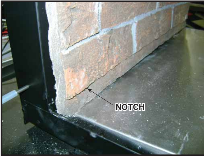
Figure 14.14 Notched End of Side Refractory
