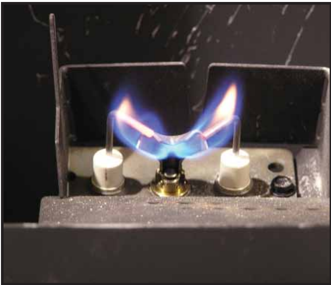
Figure 3.1 IPI Pilot Flame Patterns
