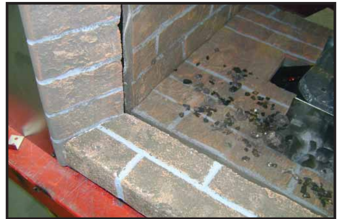
Figure 14.27 Outer Hearth Installation
