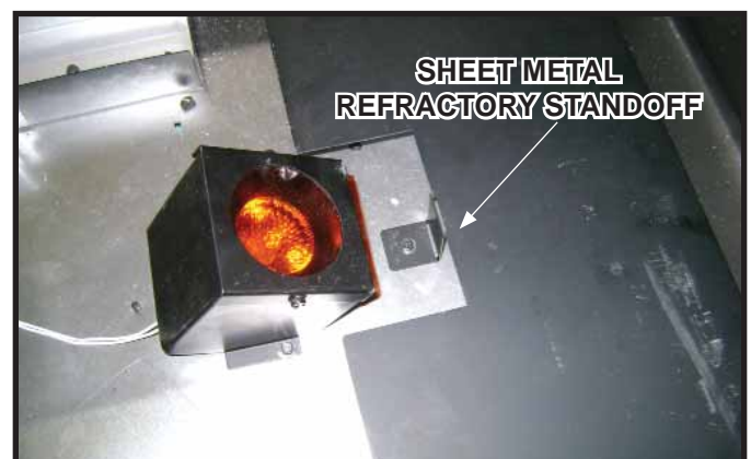
Figure 14.13 Accent Light Bulb Installation Completed
