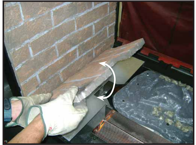
Figure 14.16 Positioning Inner Bottom Refractory
