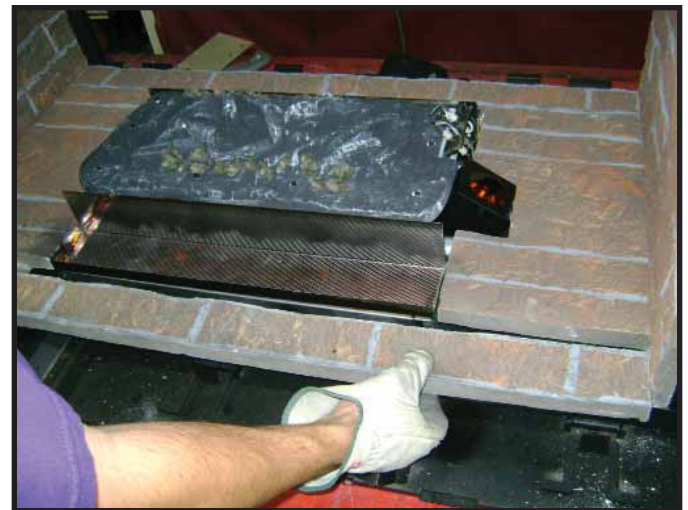
Figure 14.18 Positioning Outer Bottom Refractory.
